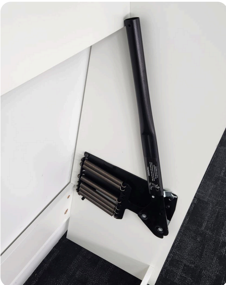
18. Tension bar fitted.
